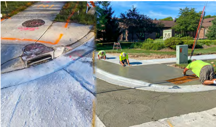
ADA-compliant ramp installation
